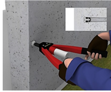
3. Rivet up to the rivet shank cutout.
